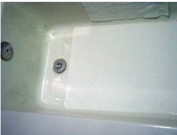
Rebuilt and Slip-Grip coated
