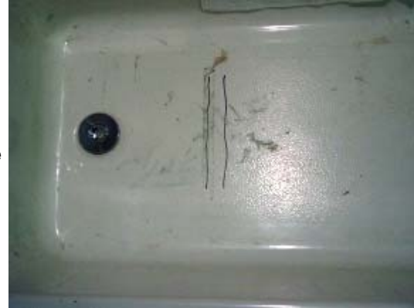
Close up of a cracked area
