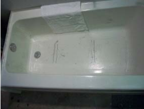
Cracked tub bottom in two locations
