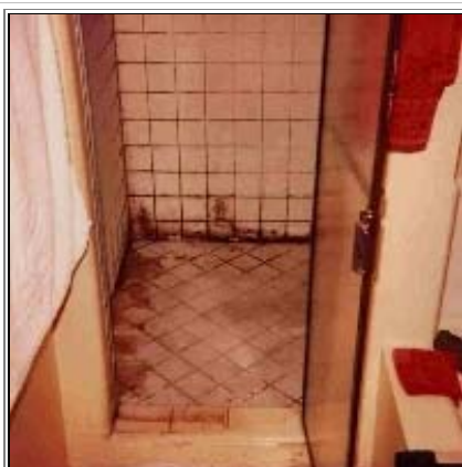
Ceramic Tile Walls & Floors
